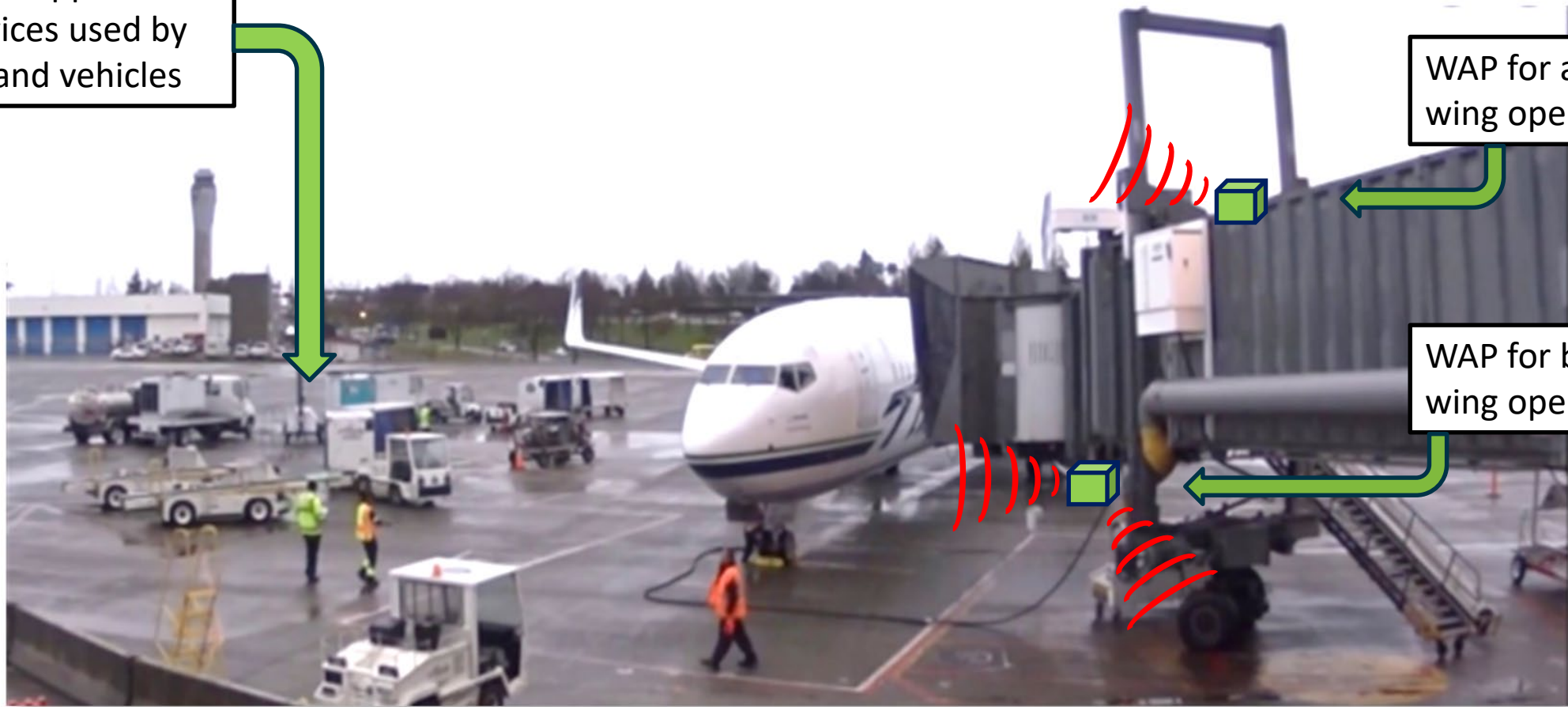
Antennas are oriented so that the signal can reach between the rear door and the tail of the aircraft where most of the Wi-Fi use will take place.
